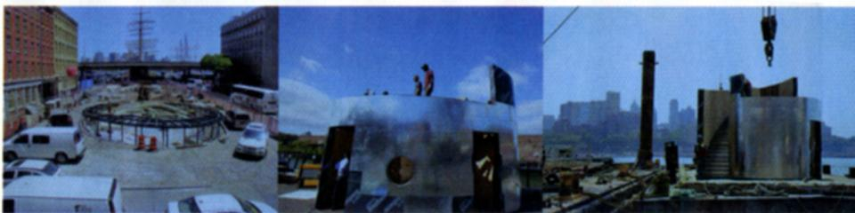
About 200 sketches later, Rockwell had outlined a site plan shaped like an infinity symbol. It contains the Aquatheater, a series of wading pools; the Listening Forest and the larger Whispering Forest, both built from red-painted cast-iron pipe; and the Crow's Nest, a red-painted steel cylinder with stairs curving up to a lookout platform. Squishy green matting, which flows around the Crow's Nest and the two Forests, is said to be Mayor Michael Bloomberg's favorite part. —*Nicholas Tamarin*
